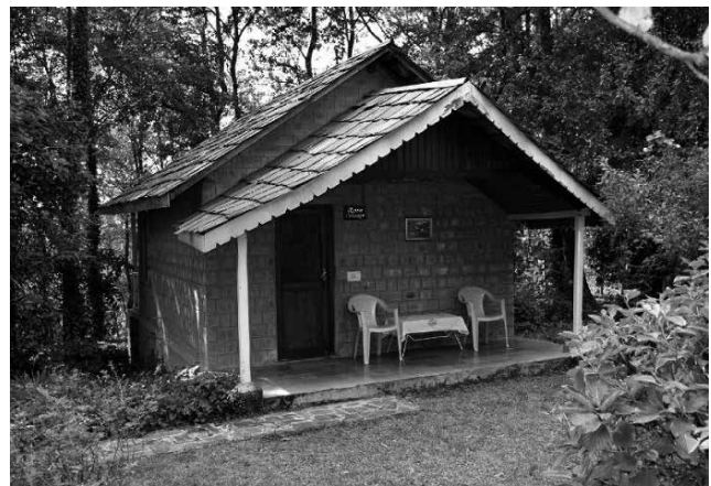
Figure 3(b): Country Cottage at Palampur, Kangra
