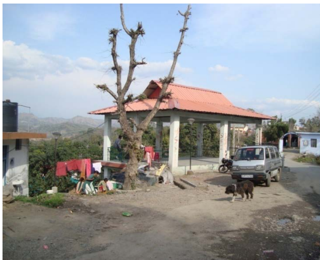
Poor Roads Condition in Baroh
