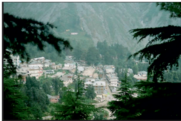
Figure 4 Structures in the Dharamkot area in Dharamshala, Himachal Pradesh, India
