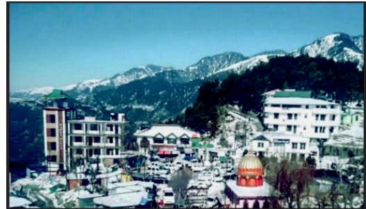
Figure 7 Hotel Buildings in the Naddi area in Dharamshala, Himachal Pradesh, India
